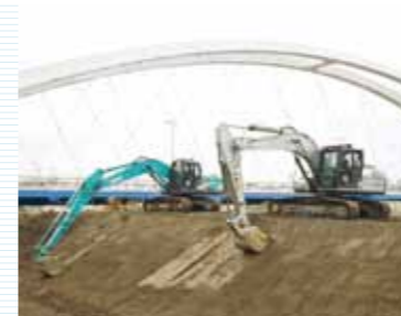
Hybrid excavator (SK200H) in operation
